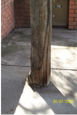
Power pole at Club house needs replacing and repositioning to side of building
