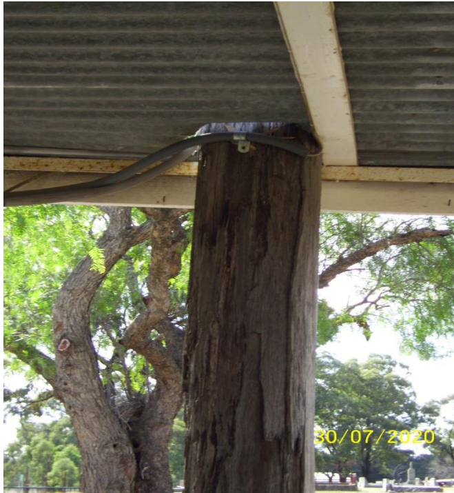
Power pole at Club house needs replacing and repositioning to side of building
