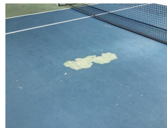
Tennis court surface delamination
