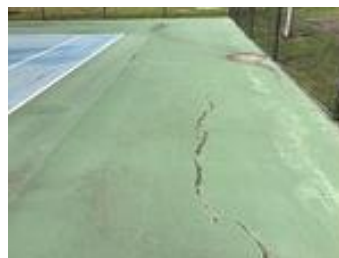
Tennis court surface cracking
