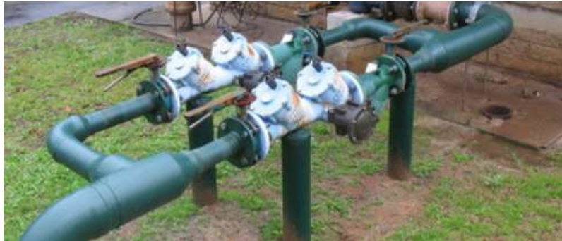
Image: Fire Service Backflow Device
