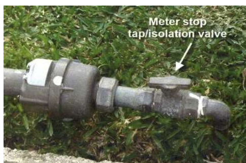
Figure: Meter stop tap or isolation valve
