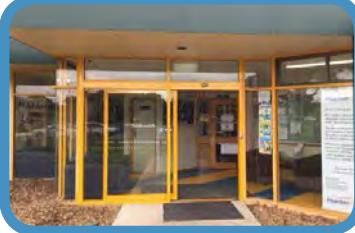
The OOSH building has a new automatic front door. This door is compliant with Australian Standards for access. OOSH also had a wider doorway directly into the classroom installed to be compliant with AS1428. Disability access has vastly improved with many comments from families on how easy it is to get their strollers through each doorway.
