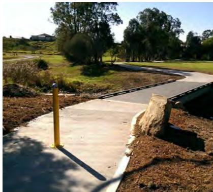
Repairs have been undertaken to a number of areas within the cycleway network. A link from Acacia Circuit to Wattle Ponds Road through Allan Bull Reserve has been established. This has included the construction of a pedestrian bridge crossing and approximately 270 metres of new concrete cycleway. These works have continued to expand the off-road linkages for the community.
